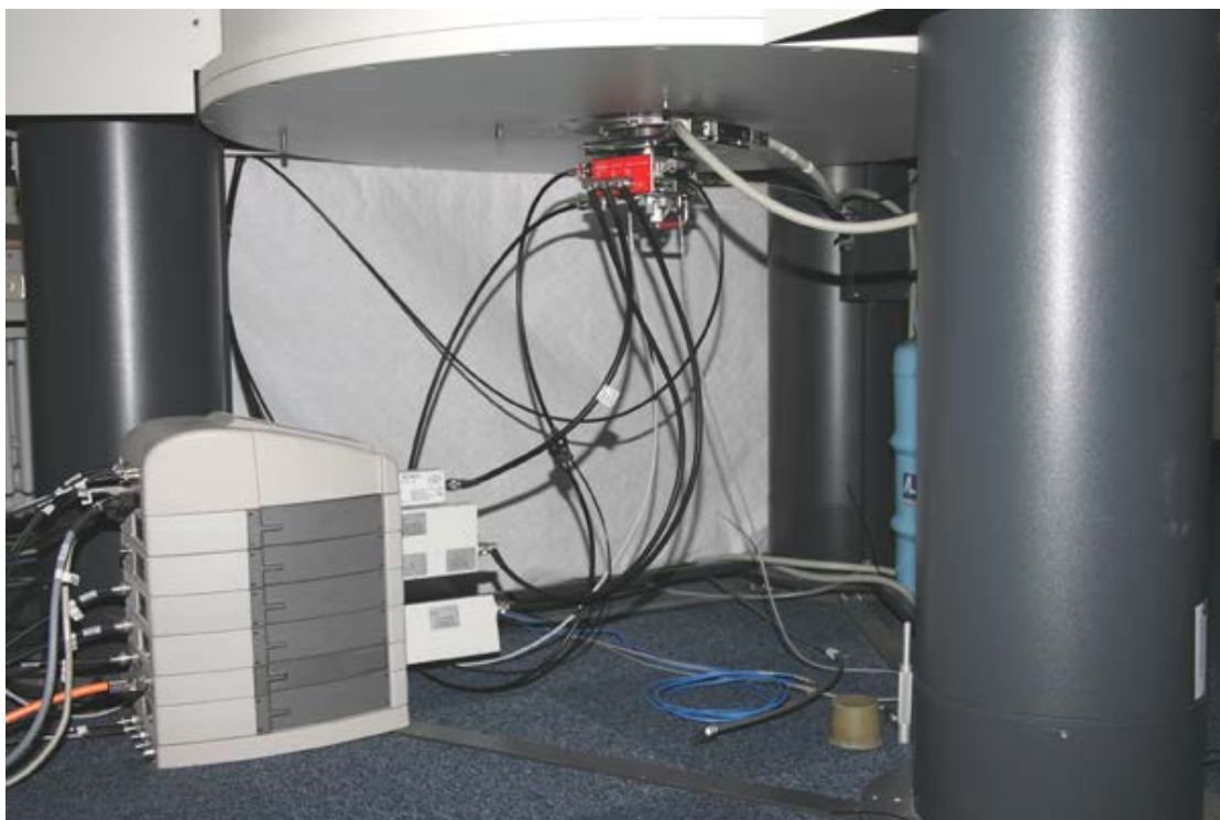
Figure 3.40: Example of a 600 WB NMR Instrument Site
